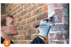
Stormdry can be applied by brush around details such as windows. Care should be taken to ensure that Stormdry does not splash onto glass, paintwork, plants, etc. Any splashes should be cleaned away with warm soapy water.
