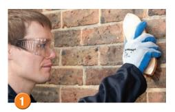
Carry out surface preparation as described in Preparation section. Remove any loose mortar, dust etc... using a masonry brush. When biological growth such as moss, algae or lichen needs to be removed, apply Soluguard Multi-Surface Biocide in accordance with instructions.
