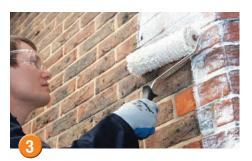
Larger areas can be covered more quickly using roller application. Stormdry can also be applied by electric roller or airless spray – call our technical department for details.
