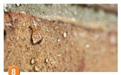
As Stormdry is formulated to penetrate deeply into masonry it can take up to two months after application for a noticeable "beading effect" to appear when rainfall strikes the wall. The masonry will be resistant to light rain after two to four hours.
