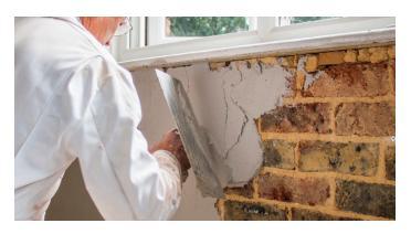
coat should be delayed. Rapid drying out of the plaster should be avoided.
